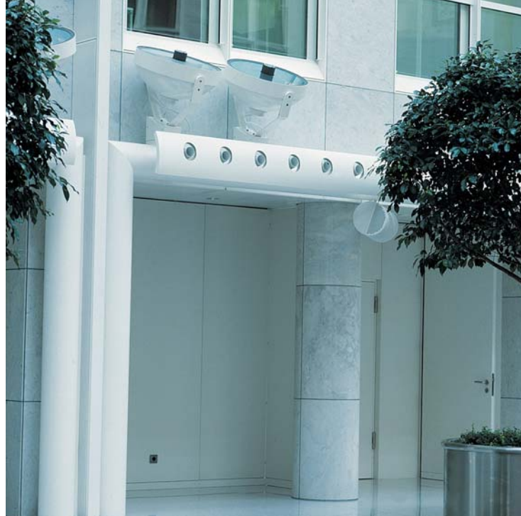
Swivel jet nozzle, type DW-V2, in the entrance hall of the Dresdner Bank AG in Frankfurt / D
