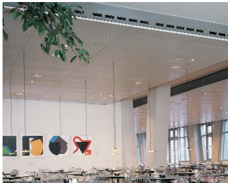
Linear whirl outlet, type WL, in the entrance hall of the insurance company 'AachenMünchener Versicherung AG' in Aachen / D
