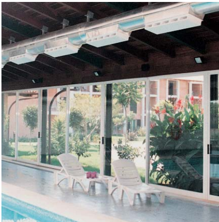
Linear whirl outlets, type WL, in the swimming pool of a hotel on Majorca / E
