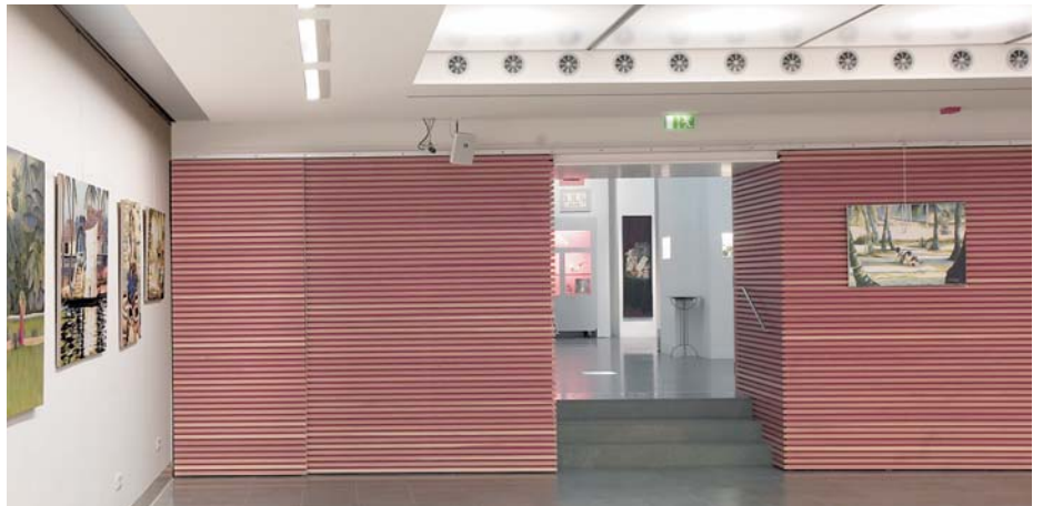
Twist outlets with sharp-edged exits, type D-NE, in the 'Art Cult Center' museum, Vienna / A
