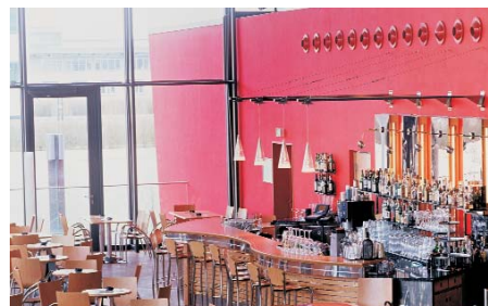
Swivel jet nozzle, type DW-V2, in the restaurant of the multiplex 'Filmpalast-am-ZKM' in Karlsruhe / D
