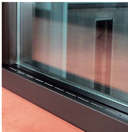
Window air curtain unit, type FSG, in an office of the Dresdner Bank AG in Frankfurt am Main / D
