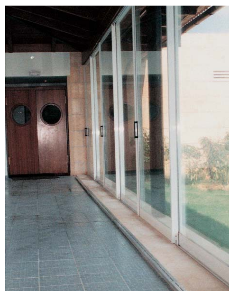
Window air curtain unit, type FSG, in a hotel on Majorca / E
