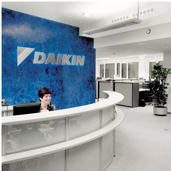
Multiplex outlets, type FA-VT in single-row design, in the entrance area of 'Daikin Airconditioning Central Europe Handels-GmbH', Brunn / A
