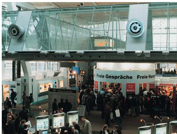
Swivel jet outlets, type SW, in the glass supply air duct, Hall 26, at Hanover Fairgrounds / D
